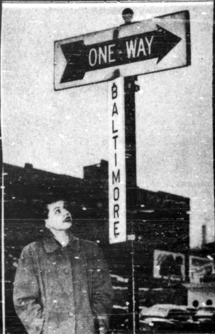
NEW STREET NAME SIGNS were placed on Baltimore avenue yesterday from Ninth to Fourteenth streets. The signs were mounted vertical to the pole and lower than the former signs to enable motorists to read them easier. Miss Doris Brockman, 21, of 419 East Thirty-sixth street, is shown looking at one of the new signs on the northwest corner of Fourteenth and Baltimore. The signs are painted with a reflecting paint background to give added visibility at night. If motorists react favorably to the signs, the city plans to mark other downtown streets in a similar manner. —(Kansas City Star photograph).
