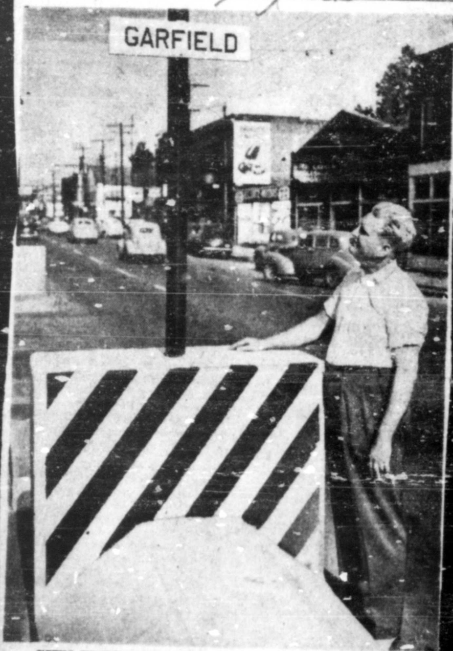
CITY EMPLOYEES HAVE STARTED ERECTING new street signs on the safety island light poles on Fifteenth street. The new signs are of wood with a white background and the names lettered in black. T. J. Seburn, city traffic engineer, said the additional signs would aid motorists because of the width of the street. Frank Ramel, a used car dealer, is shown viewing one of the new signs—(Kansas City Star photograph).
